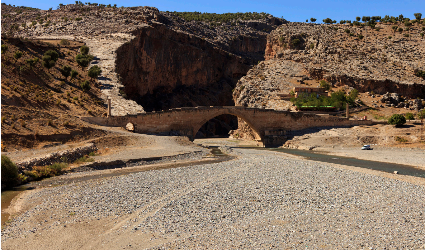
Ancient Cendere bridge built during Roman era over the Euphrates, now largely dried up | mehmetakgul | Getty Images
